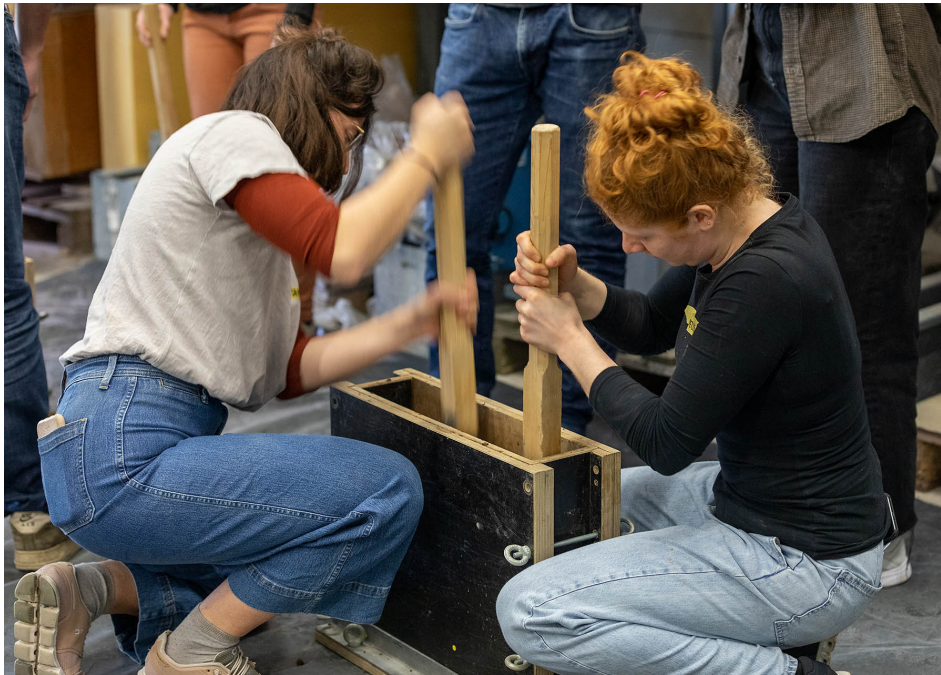
03 Rammed earth: compacting earth in layers. HSLU 2023 materials workshop
